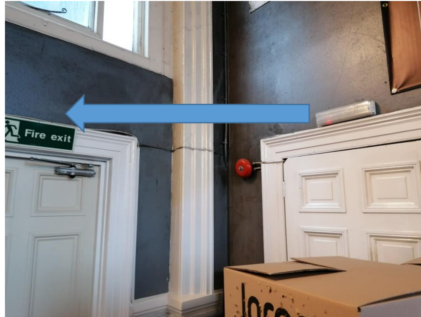
Re-locate emergency light
