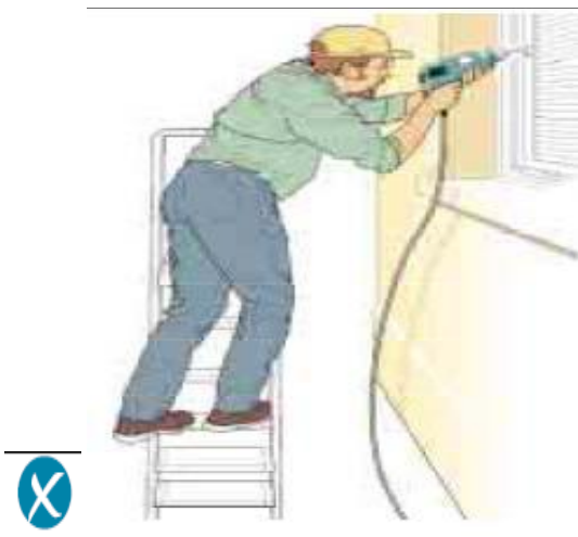
Incorrect – steps side on to work activity
