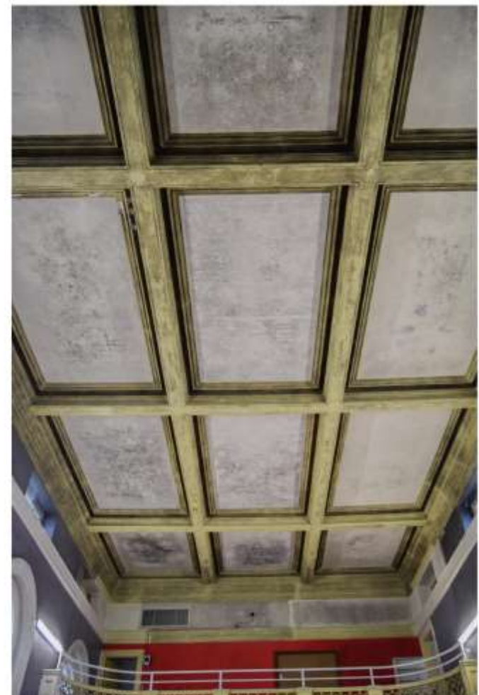
v) [above] coffered and moulded ceiling showing cornice and clerestory windows
