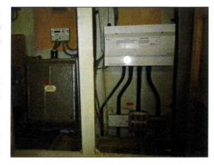
Parts of the installation are dated. As such, we consider that a NICEIC qualified engineer should carry out a functional test and advise on any upgrading works for obvious safety reasons unless the installation has been examined and tested within the last five years.
