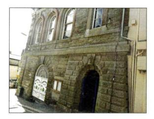
Feature granite archways to two ground floor openings. Granite work generally sound with a feature granite buttress adjoining the main entrance door. However, the granite keystone above the entrance door was noted to be slightly cracked.
