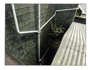
There is no rainwater gutter to the sloping slate roof cover to the west to the stairway.
