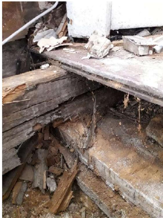
Further investigation is needed on the condition of the floor joists and woodwork in the Mayors Parlour. The sash window in the Members' Room is also partially rotten and will require repair.
