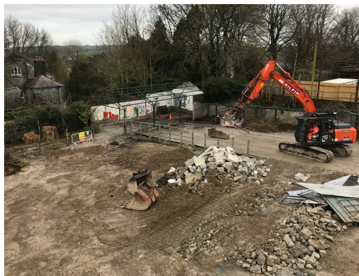
Demolition in January 2021
