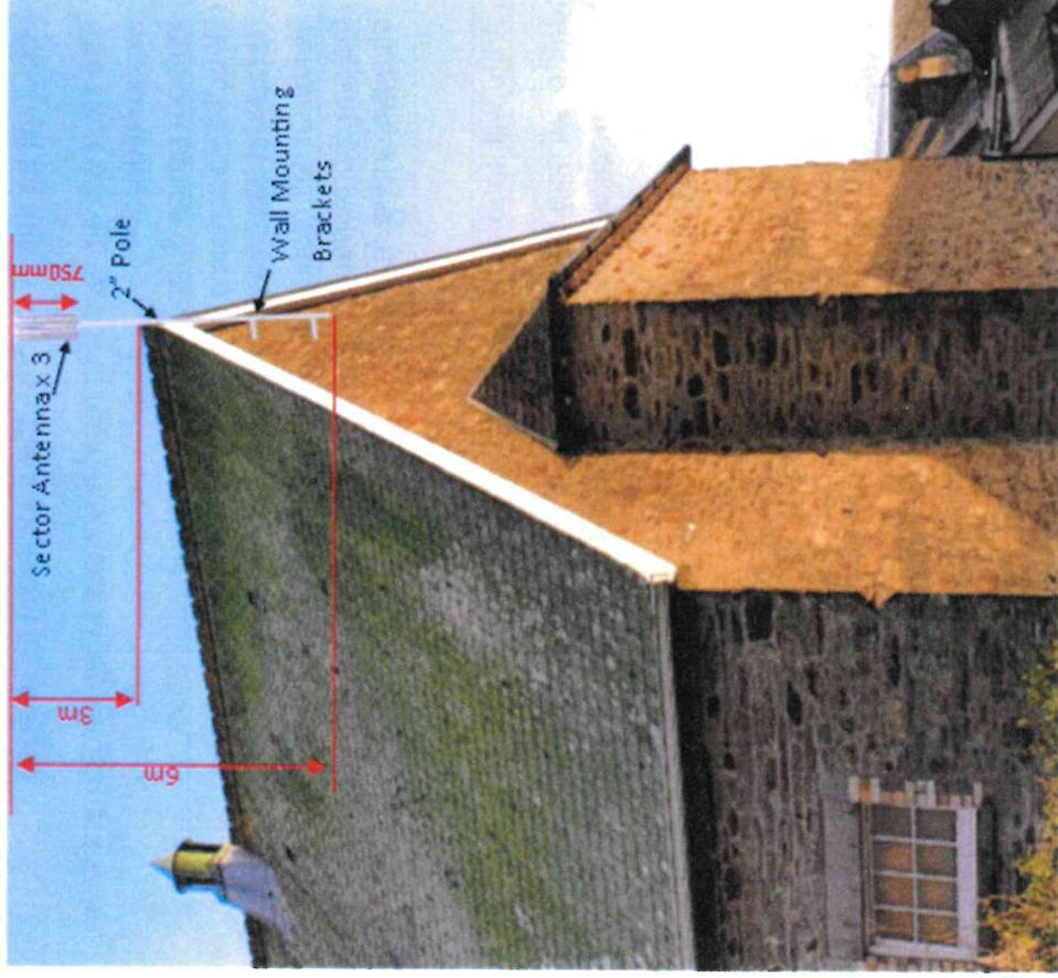
The radio equipment will be fitted to a pole that will extend approximately 2.5m-3m above the pitch of the building.
